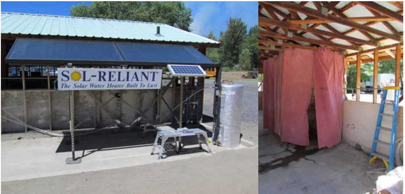
Contractors come for continuing education credits about solar hotwater from Mr. Sun Solar and attendees get to try out the resulting showers! Credit Dave Felley
